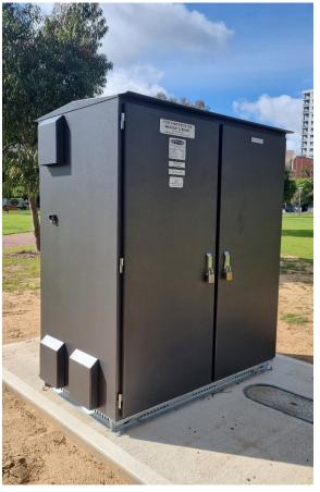
The Light Square Electrical Major Switch Board was upgraded to facilitate a 300amp supply to the area. This upgrade will support events such as Fringe and Illuminate in this space and potentially increase revenue.
