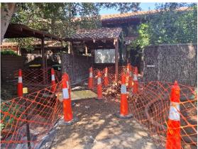
Photos show excavation was undertaken using a mechanical and hydrovac process due to the large number of services and protection of tree roots.
