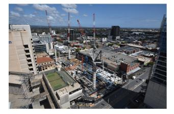
In the last quarter, major progress has continued on site including the completion of the basement excavation and retention works to the lower basement levels. This has involved the removal of 83,000 tonnes of soil material from site in total.
